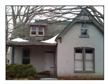
What was once a great example of Gothic Revival architecture has become a worsening eyesore. The house, which features a high pitched gable roof and ornamental brackets, is slowly succumbing to structural failures in the roof, walls, porch, and rear addition. Its condition is severe enough that it could be considered a "demolition by neglect". (On Endangered Buildings List since 2015)
